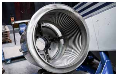
Preparation for welding the external protective cover
